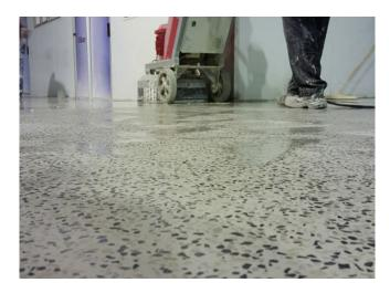
Polyscreed PMC Terrazzo is a ready to use blend of hard wearing marble chip aggregate, polymer modified cement and additives which produces an abrasion resistant, impact resistant, 8 - 10 mm floor overlay system.
