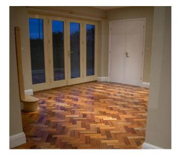
An easy to use, acid catalyzed conversion varnish based on a blend of alkyd-amino resins used in semicommercial environments. Produces a highly attractive and functional finish.
