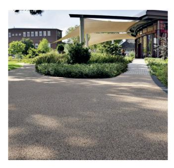
Elastopave is a surface covering system where selected graded aggregates are mixed with a PU resin binder and placed by trowel onto a prepared surface to yield a seamless, strong, durable and attractive surface.
