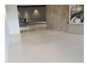
Polyscreed Earth Flow is a flow applied high performance, high early strength, decorative, self-levelling floor system applied at a nominal thickness of 4 mm.
