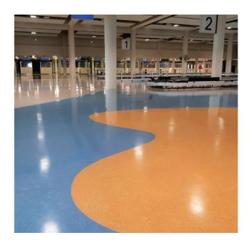
A decorative, hygienic, epoxy resin based terrazzo floor finishing screed. Exhibiting an exposed aggregate texture with a smooth surface of uniform colour designed for excellent resistance to abrasion, chemical attack and other physical aggression.
