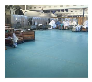
A high performance three component polyurethane roller coat resin system providing exceptional physical and chemical resistance in demanding industrial environments. Designed for coating of concrete, existing polyurethane screeds and covings.
