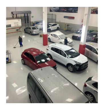
Solidflow SL 1000 is a three component, solventfree, self-levelling epoxy system applied at a nominal thickness of 1 mm.
