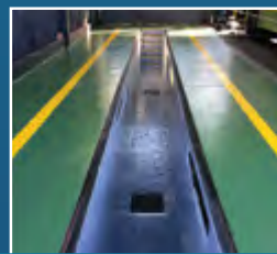
Polyurethane floor coatings
