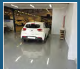
Epoxy self-levelling screeds
