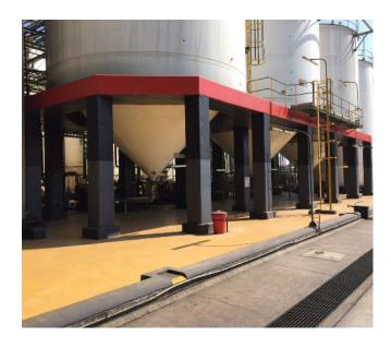
Chemical resistant, 100% solids blend of selected Novalac epoxy resins cured with a high cross-linking activator specifically formulated for coating, laminating or lining steel tanks, concrete bunds and other surfaces in heavy duty acid or highly alkaline environments.
